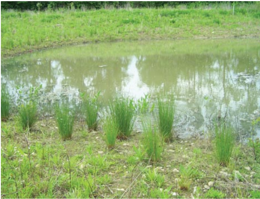
For the West Chester bioretention ponds, the budget drove the design. The budget was divided between earthwork, water-control structures, vegetation, and design.
