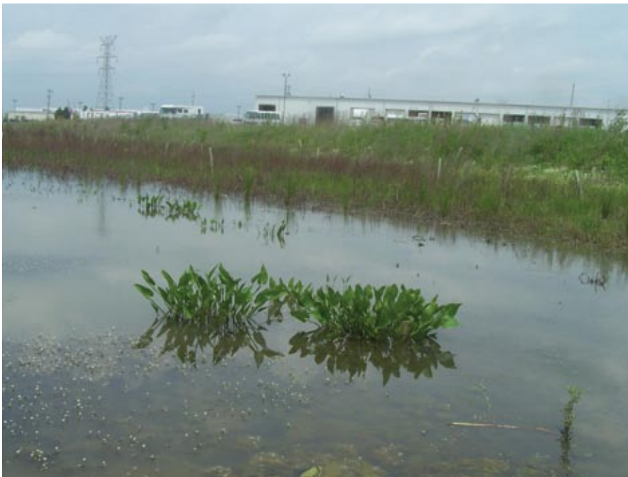
The bioretention ponds are functioning as expected. Post-construction water-quality monitoring has begun, and vegetative survival is also being monitored.
